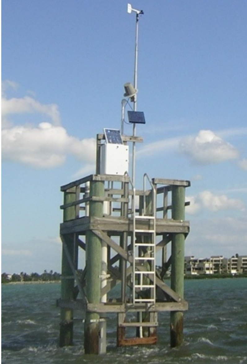
Figure D-17: Florida Department of Natural Resources water quality station
